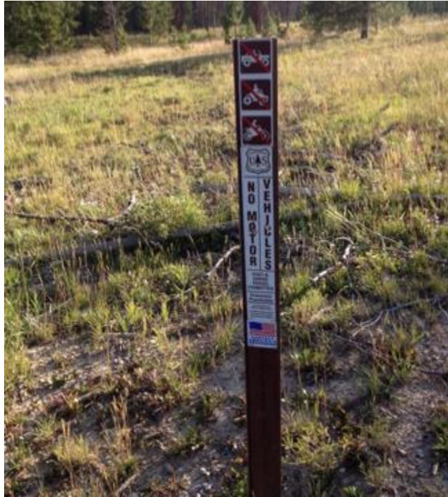
Picture 12. Example of effective signage on carsonite sign on an older user-created route. Carsonite signs were observed to be effective on several older or user-created routes, but should not be considered an effective closure or signing method for well-established unauthorized roads.
