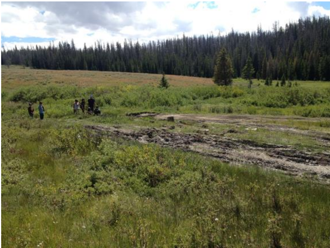
Picture 16. Example of SRNM, maintenance needs results in unauthorized parallel routes.
